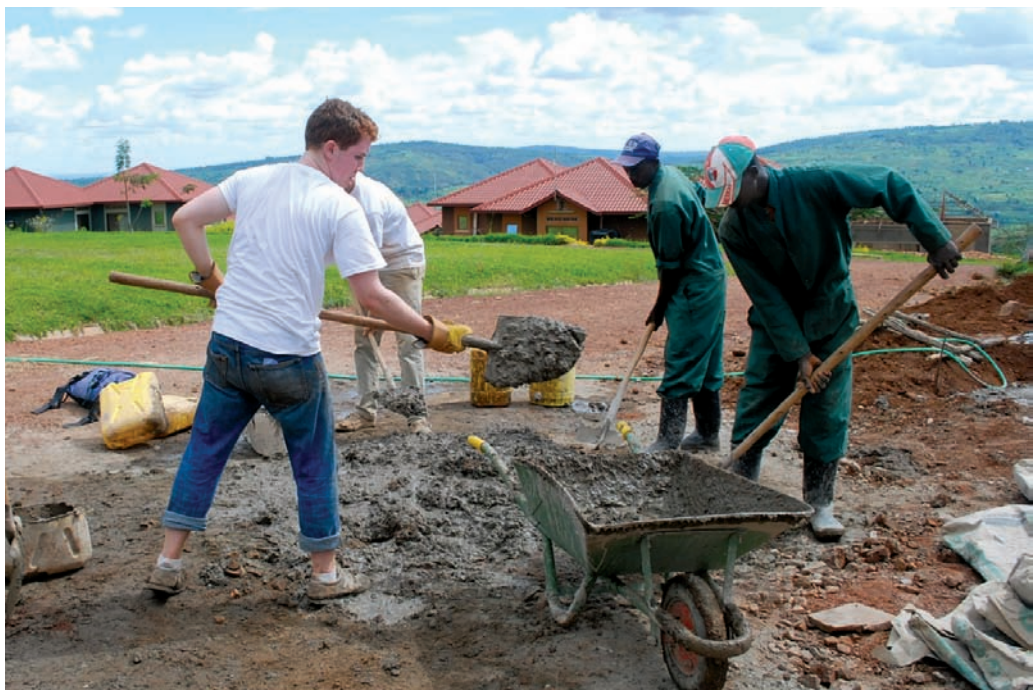
John Plaisted helps mix concrete to construct benches and tables for a gathering area outside the student canteen.
