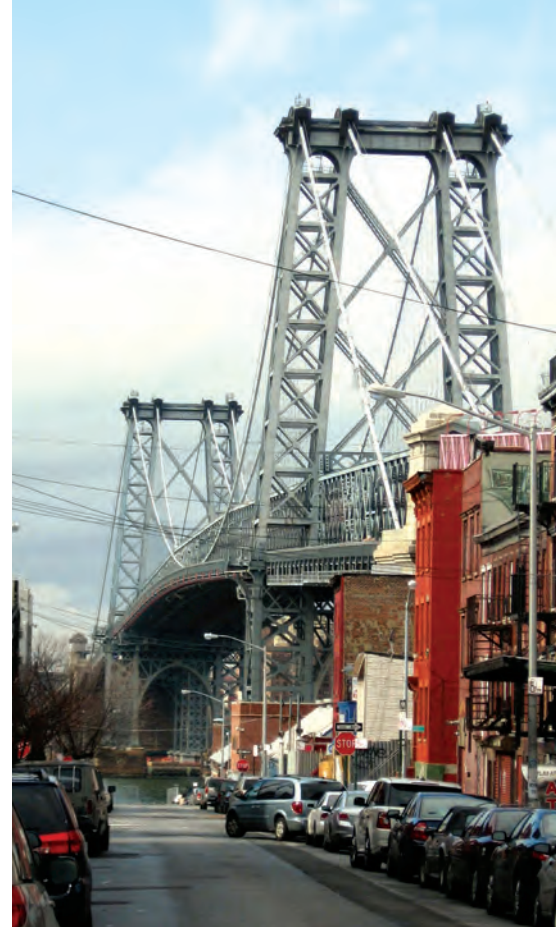
The Williamsburg Bridge: Rehab, not rebuild.
